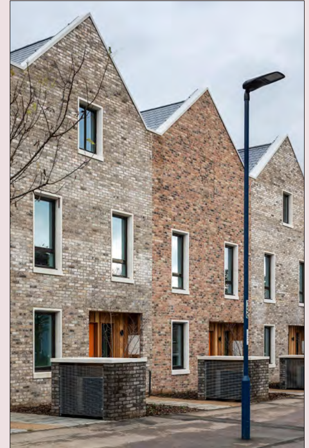
Above: Integrated refuse stores at the front of homes keeps the street neat and tidy.
